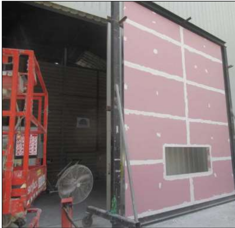
Picture 1: Base wall prior to installation.
