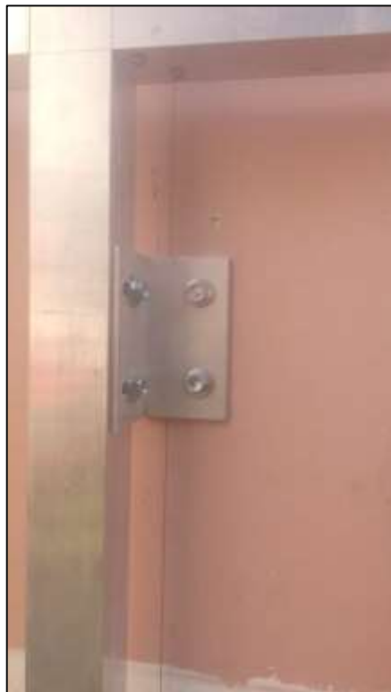
Picture 2: The wall bracket fixed onto the base wall and runners to the wall bracket.
