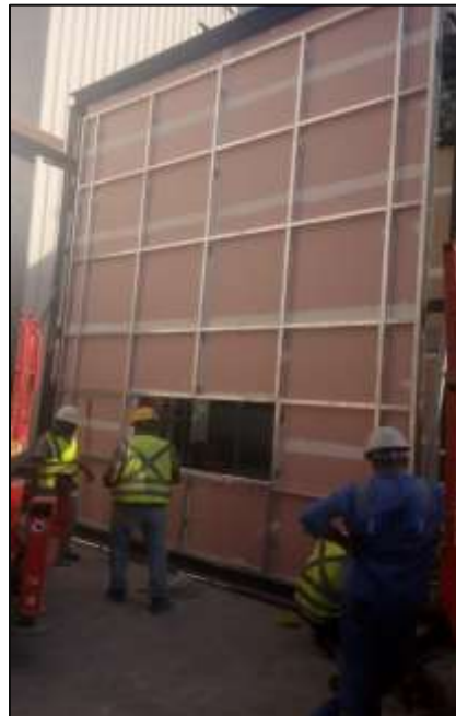
Picture 3: The runners fixed onto the wall brackets.
